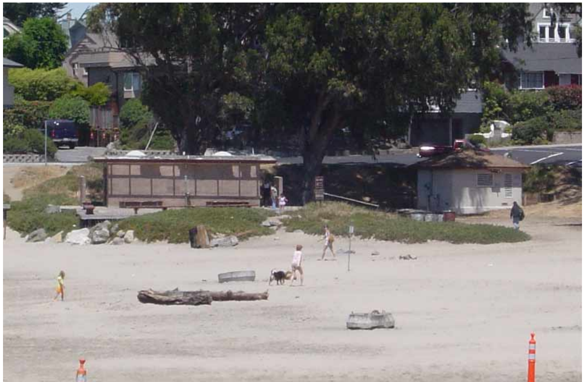
View of existing buildings on site at Twin Lakes State beach
